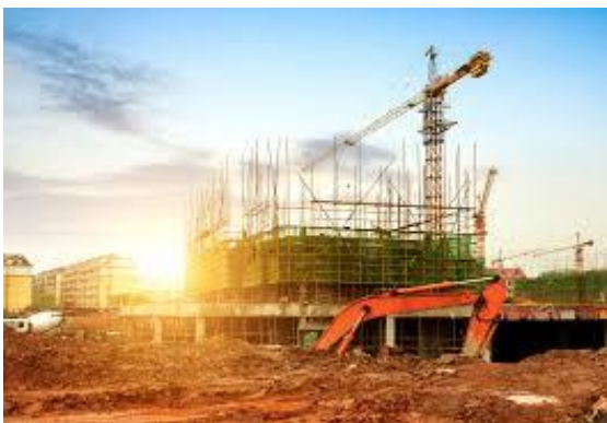
Building an office building
